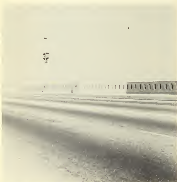
FIGURE 5. Repaired section of railing, Sixth Street Bridge, Los Angeles.
